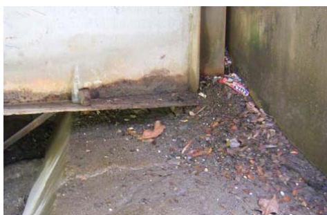
Photo 2-6 Mud, Debris & Sand on Bearing
