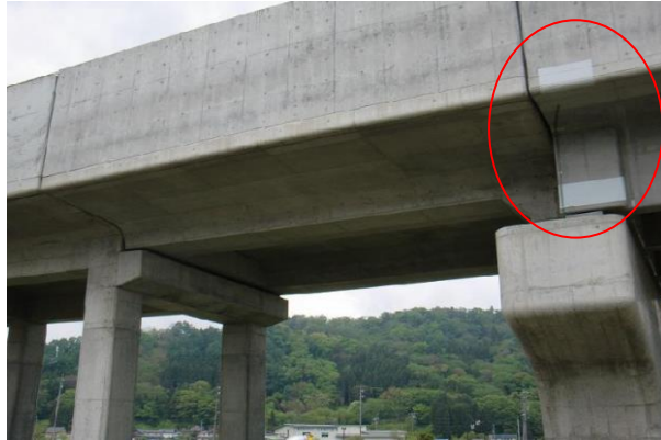
Photo 5-5 Protective Coating applied on Surface of Superstructure
