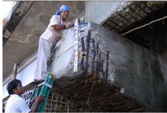
Photo 6-1 Damaged Pier for Repair by Recasting
