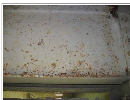
Affected surface area is 10 to 20% in a member
