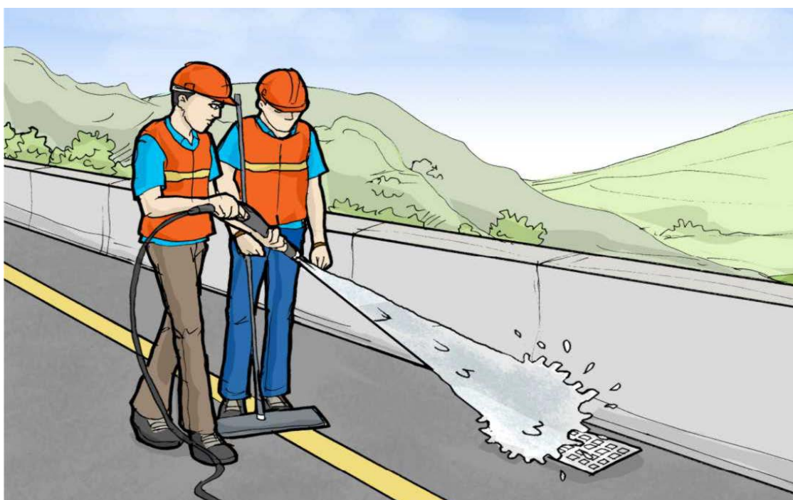
Illustration 2-2 Cleaning of the Deck Slab and its Drainage Inlet
