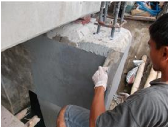
Photo 6-3 Protective Mortar applied on Substructure Surface
