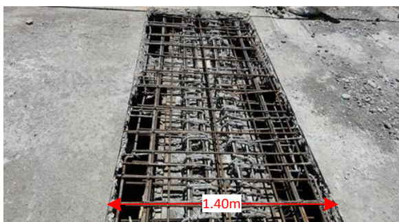
Photo 4-4 Rebar for Continued Deck Slab
