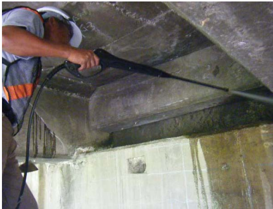
Photo 2-1 Cleaning of Bearing
