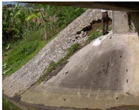
Photo 10-3 Damaged Slope Protection
