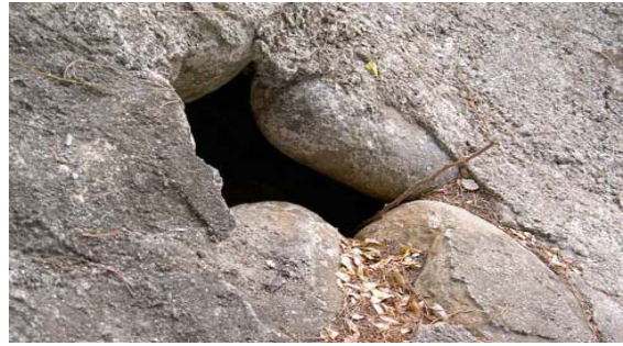
Photo 2-14 Missing Stone on Wet Masonry
