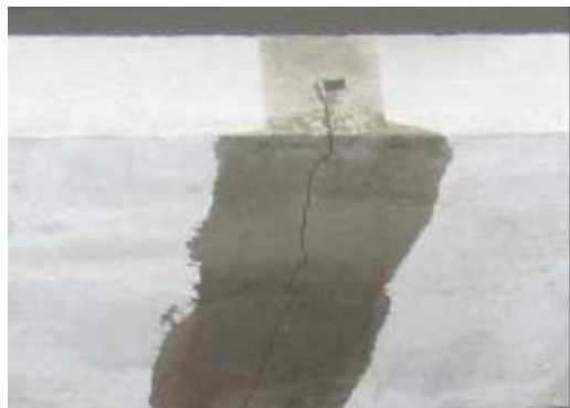
Photo 2-11 Epoxy Coating Penetrating into the Crack
