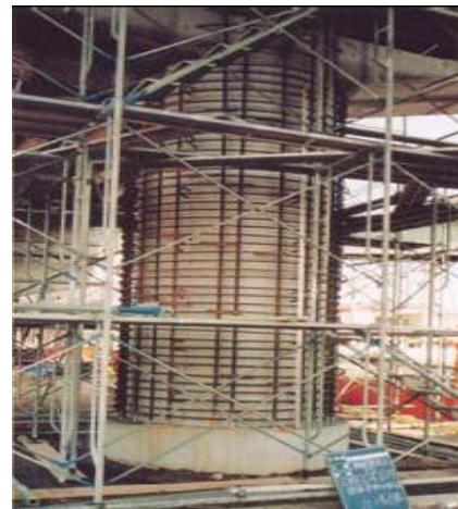
Photo 6-2 Concrete Jacket for Repair Pier
