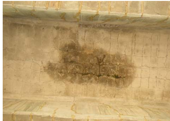
Photo 4-1 Severely Damaged Deck Slab
