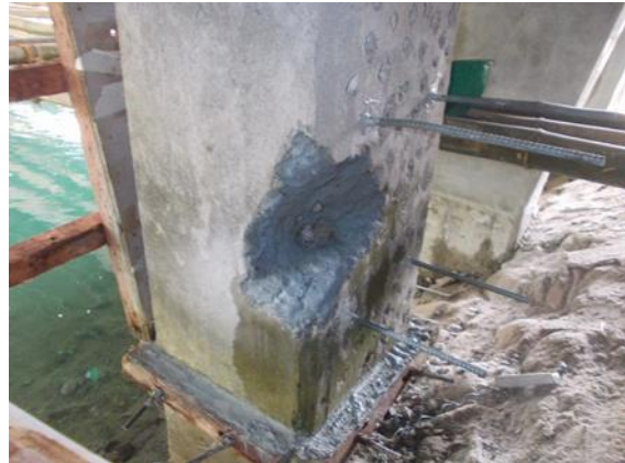
Photo 6-4 Protective Mortar applied on Patching Surface
