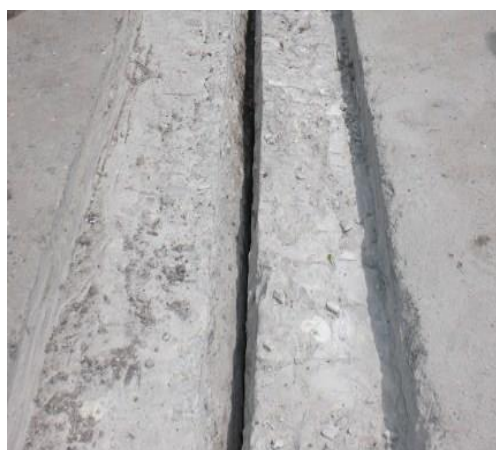
Photo 8-1 Cleaning of the gap
