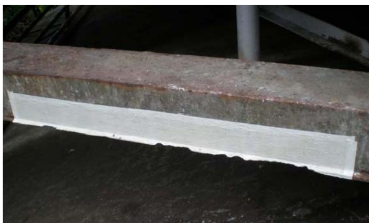
Photo 2-9 Touch-up Paint to Corroded Portion
