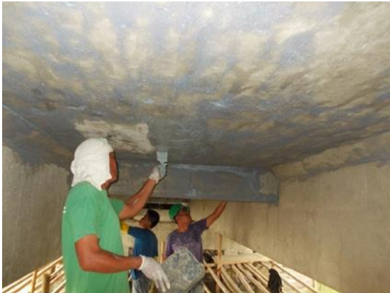
Photo 4-6 Protective Mortar applied on Deck Slab Bottom Surface
