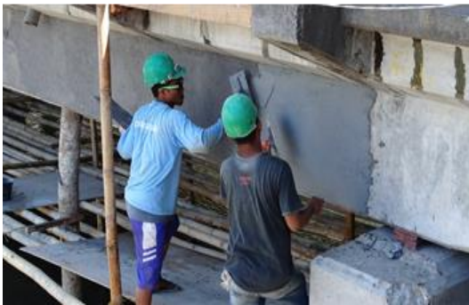
Photo 5-3 Protective Mortar applied on Girder Surface
