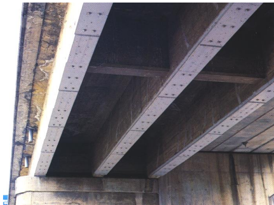
Figure 5-11 Repair of Concrete Girder by Steel Plate Bonding
