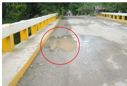
Photo 2-5 Ponding Water on the Deck
