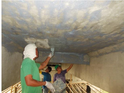
Photo 4.8 – Protective Coating applied on Deck Slab Bottom Surface
