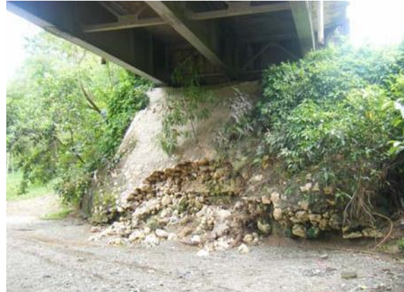
Photo 10-1 Broken Slope Protection
