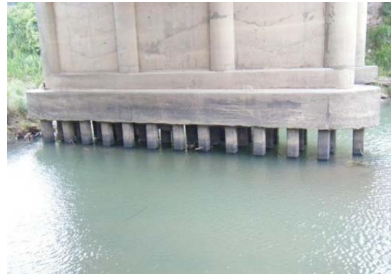
Photo 3-1 Exposed Concrete Piles
