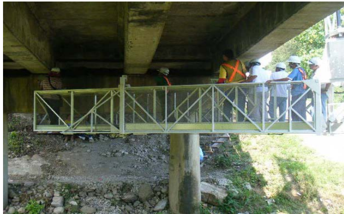
Photo 2-12 Patching Repair using Inspection Vehicle
