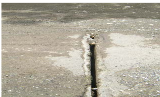
Photo 2-4 Joint is Clogged with Sand and Dust
