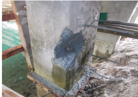
Photo 4-7 Protective Mortar applied on Patching Surface
