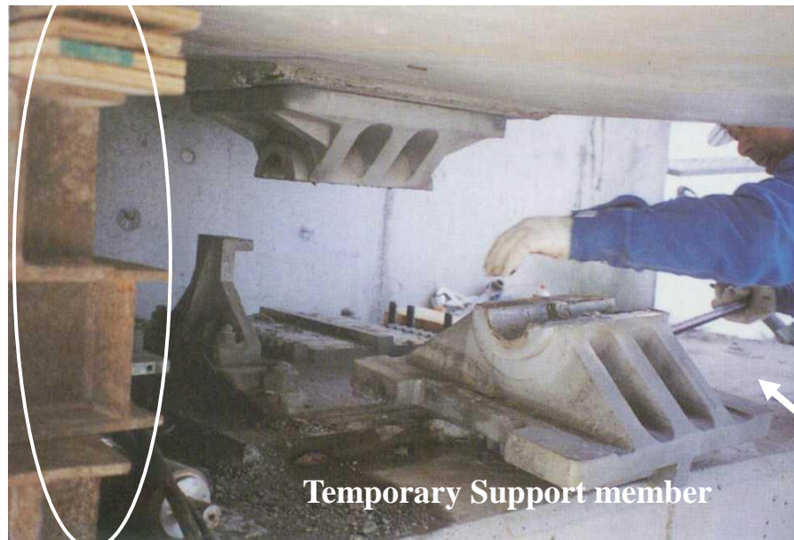
Photo 9-2 Sample of Replacement Bearing by Jack-up Girder
