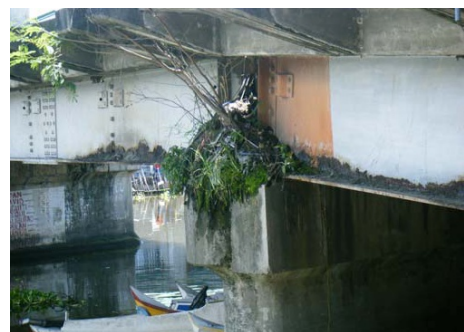
Photo 2-3 Vegetation in the Deck or Girder
