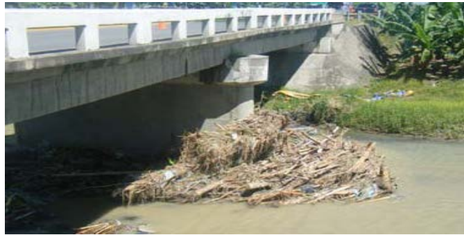
Photo 2-13 Accumulated Drift Wood and Plants around Pier
