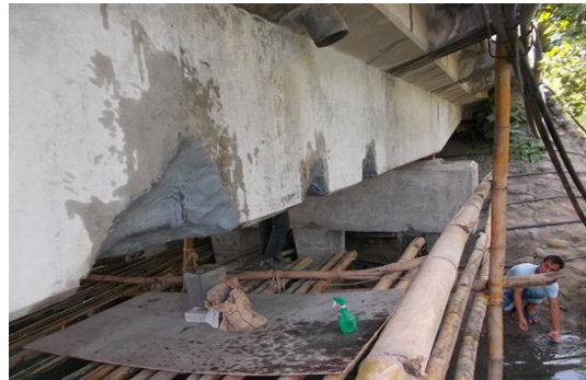
Photo 5-4 Protective Mortar applied on Patching Surface
