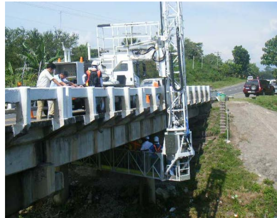
Photo 2-2 Cleaning using Inspection Vehicle
