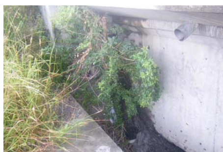
Photo 2-7 Vegetation on the Substructure
