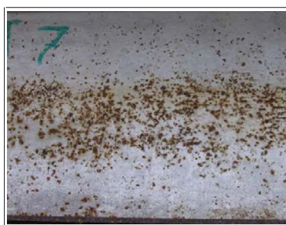
Affected surface area is 20 to 30% in a member
