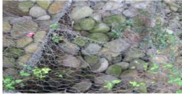
Photo 2-15 Partially Deteriorated Gabion Wire
