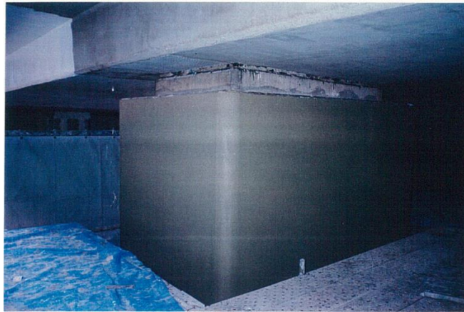
Photo 6.5 – Protective Coating applied on Substructure Surface
